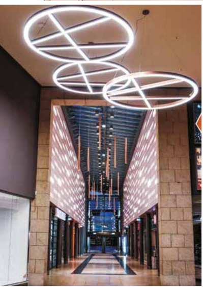
LED lighting in the Rhein-Neckar-Zentrum, Viernheim, and Billstedt-Center, Hamburg
